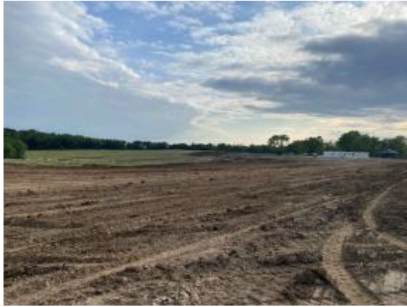
6/21 – Stripping Topsoil
