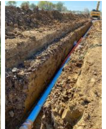
9/21 – Site Progress, Fire Mains Installed
