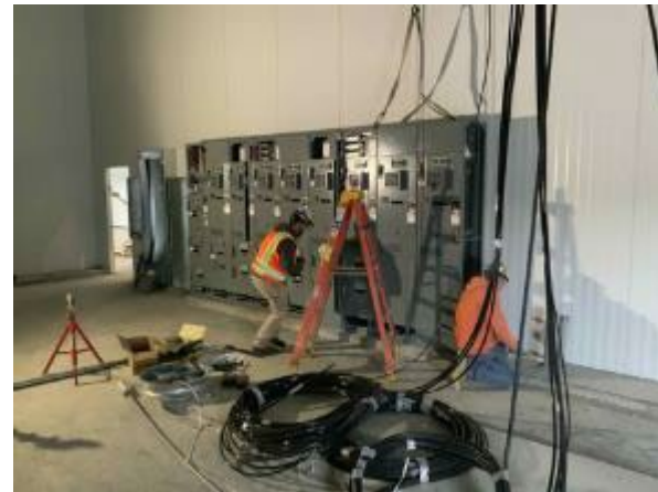
5/22: Unit 1 Interstitial, Switchgear installation, Paving, Refrigeration vessels being set
