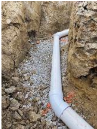
8/21 – Sanitary Drains, Building Pad Prep
