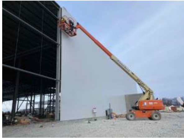
1/22: Exterior IMP, Main Cable Trays, Roofing begins
