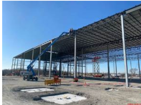
12/21 – Roof Decking going in, UG Electrical, Progress on Christmas Day!
